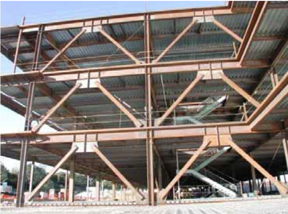
SFRS: SCBF (Specially Concentrically Braced Frame)
